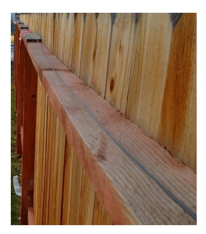
This is strung along a fence for NVIS application.
